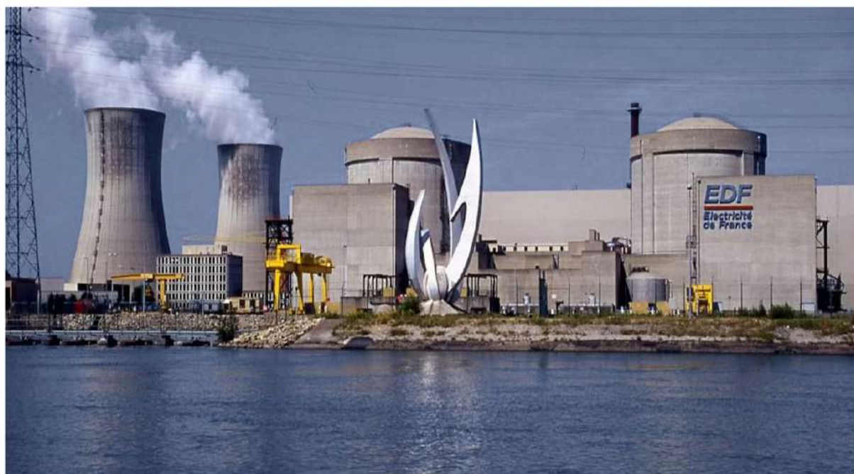
The Tricastin-1 nuclear power plant began commercial operation in December 1980. Courtesy EDF.
