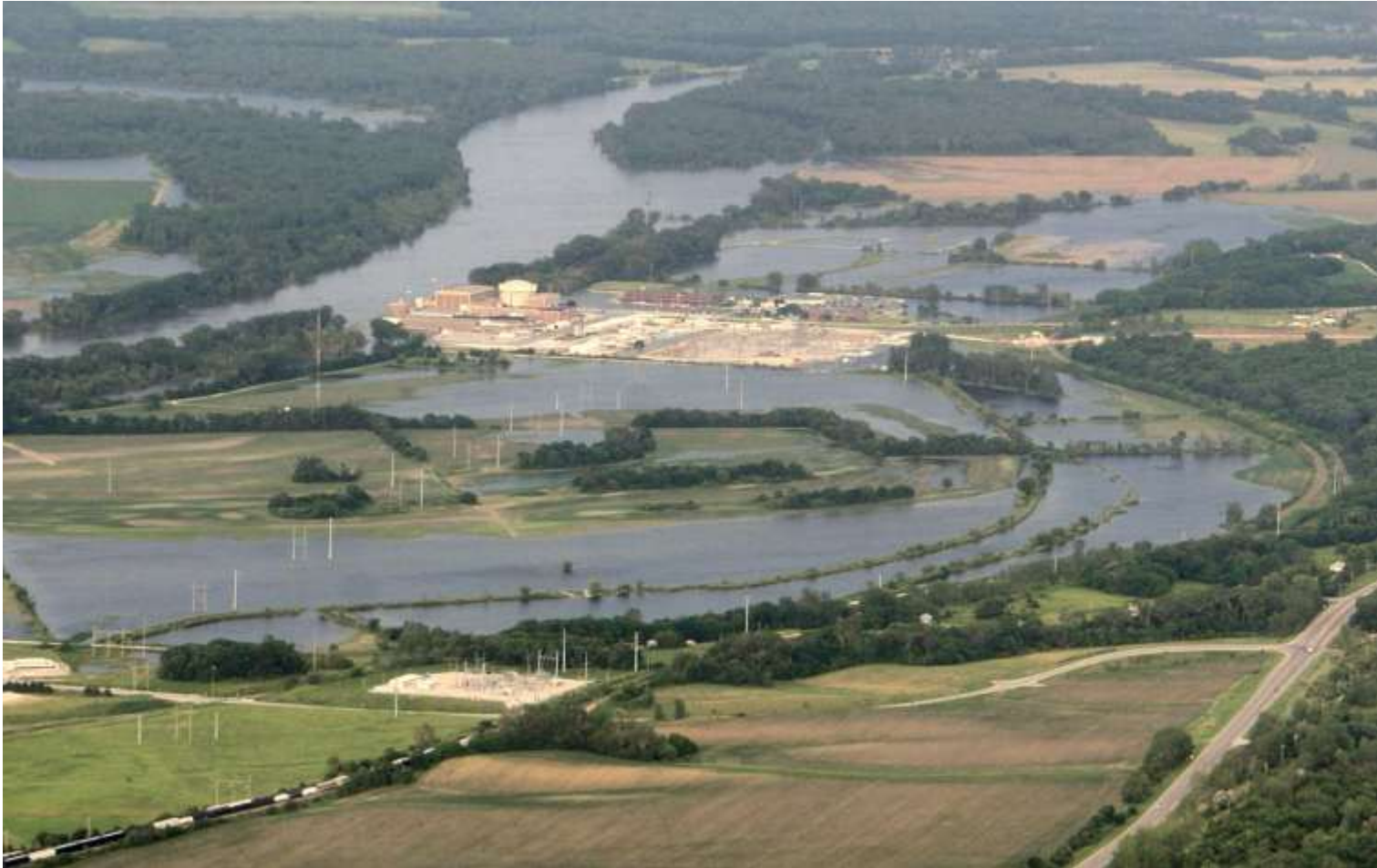
Flooding at Fort Calhoun nuclear power plant, United States, 2011.
