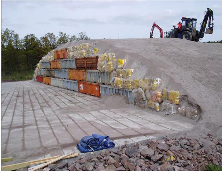
Figure 8. OKG's shallow land disposal facility at Oskarshamn.
