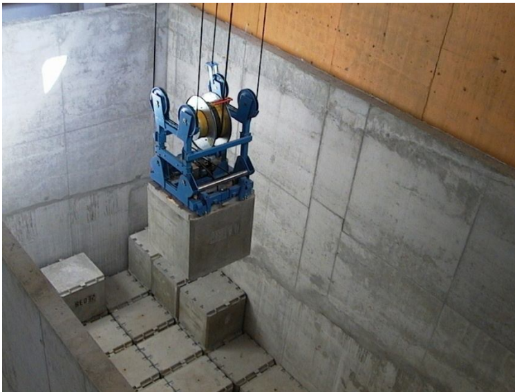
Figure 1. Radioactive waste interim storage on Paldiski site.
